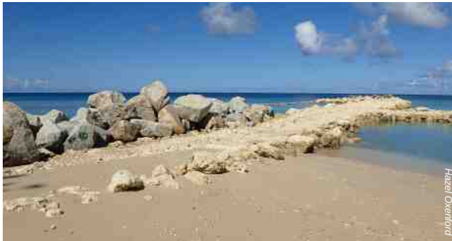
Construction of groyne at a west coast hotel
